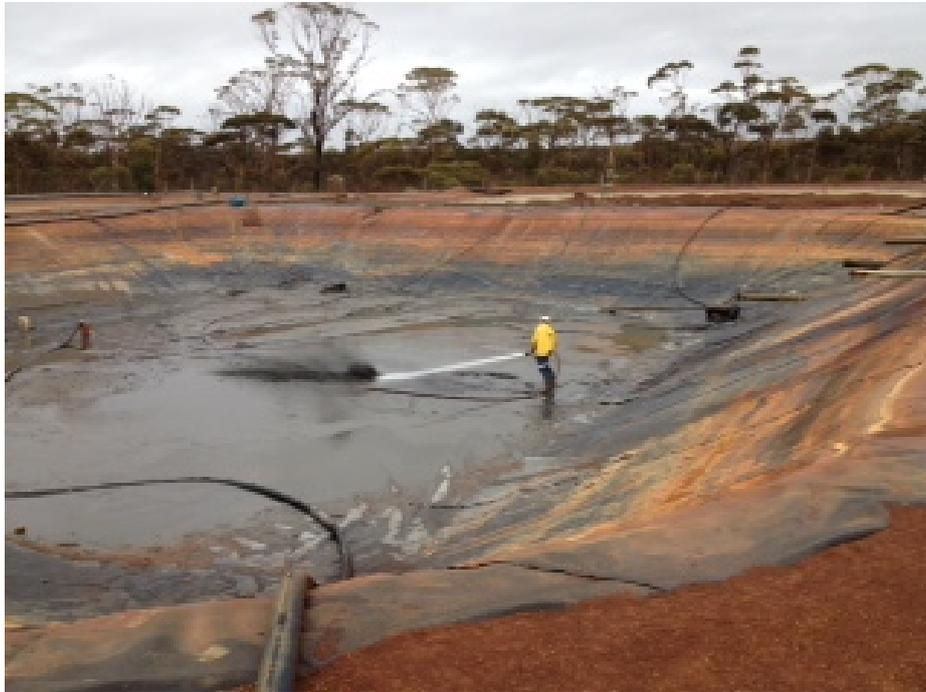
**Figure 1:** Dredging nickel concentrate from Process Water Pond 1
