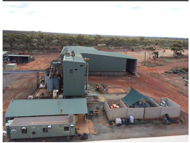
Figure 4: Black Swan concentrate shed
