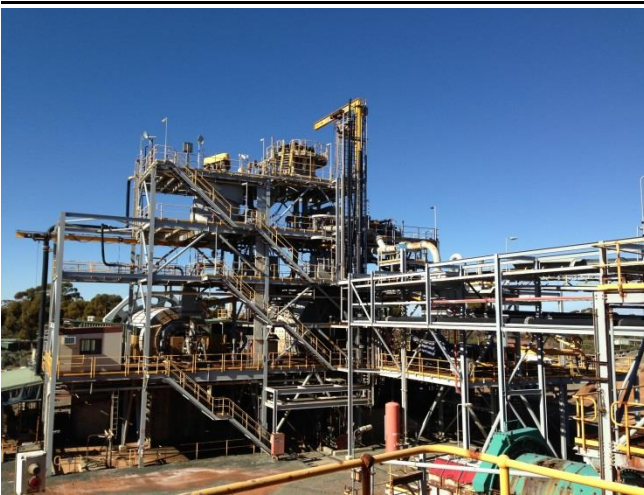
Figure 1: Black Swan processing plant
